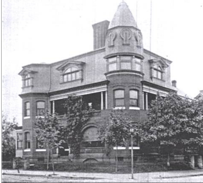
GILBERT THOMPSON'S home at Green and Vine Streets, now an apartment house, is one of the few reminders of his years in Lansdale.
