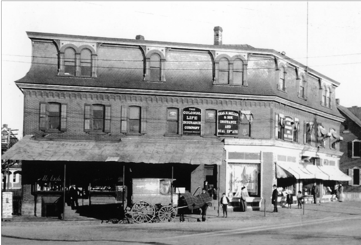
LATE 1800s VIEW OF THE ORIGINAL MOYER BUILDING
